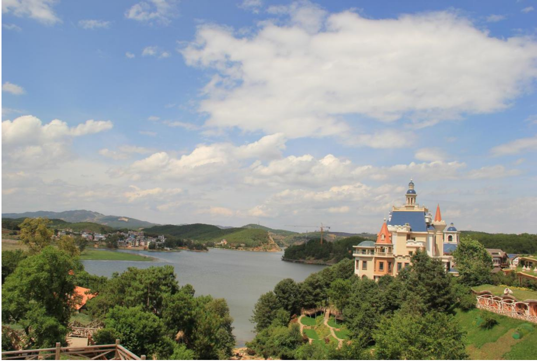
图四 项目现状图 Picture 4 Current status picture of the project
